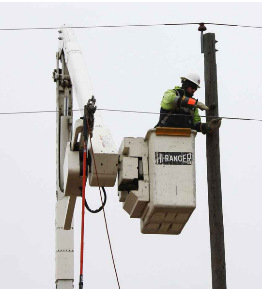
Above: Apprentice Lineman Brian Hansen repairs a broken wire tie found during spring line survey.
