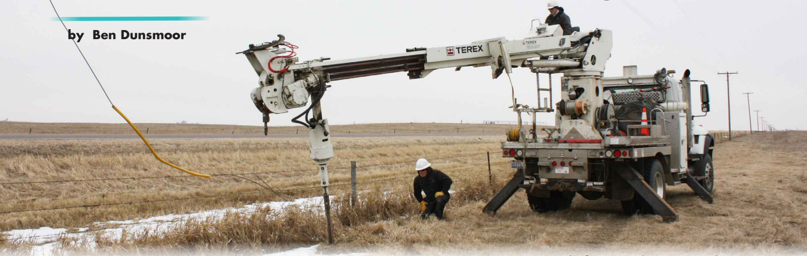
Above: Line Foreman Terry Lundberg (on truck) and Apprentice Lineman Steve Beck (kneeling) sink a new anchor into the ground to repair a guy wire.
