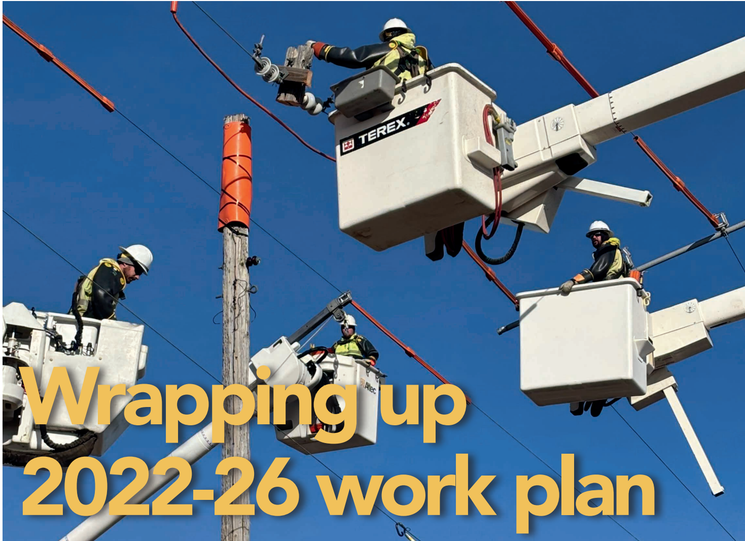
Northern Electric linemen replace crossarms on a pole earlier this year.
